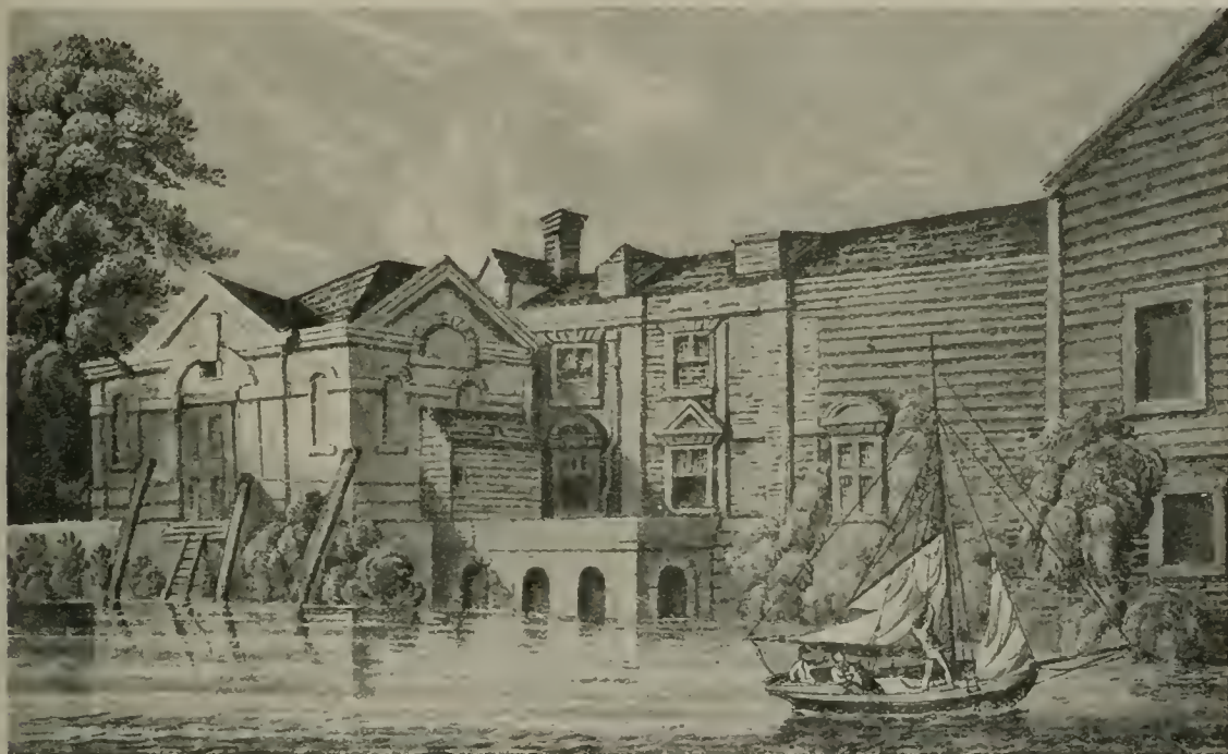
THE HOUSE ON THE RIVER AT LAMBETH CALLED GUY FAWKES' HOUSE
