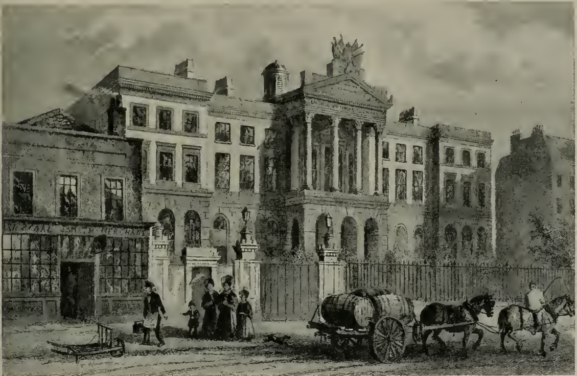
THE LICENSED VICTUALLERS' SCHOOL, KENNINGTON LANE
