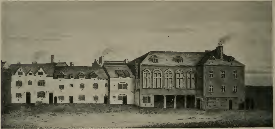
THE SOUTH FRONT OF THE NORTH SIDE OF THE MARSHALSEA PRISON, NEAR BLACKMAN STREET, SOUTHWARK
